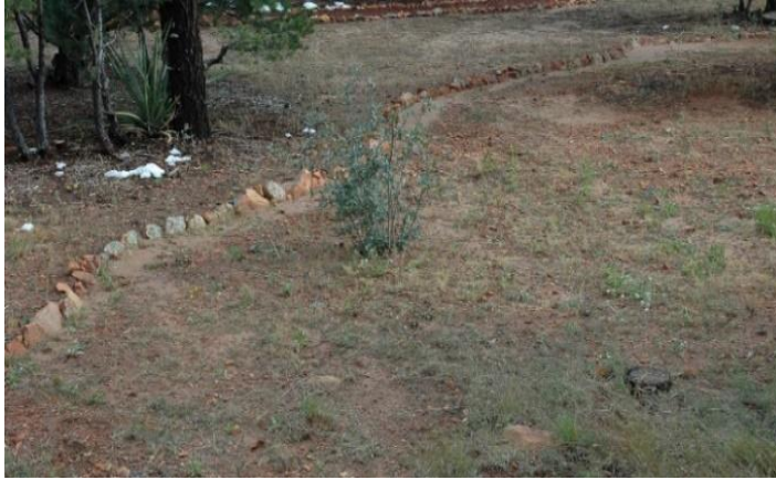
Figure 17 Short terrace wall to divert water within property
